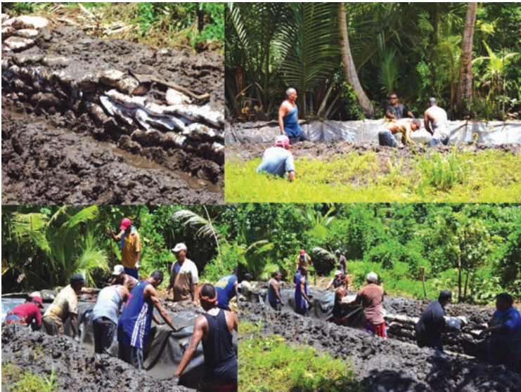
Fig. 83. Construction of the main dike with sand bags and rubber lining in Ollei, Ngarchelong
