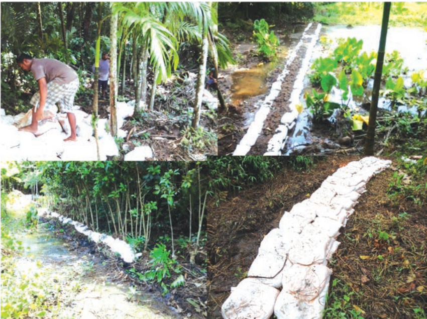
Fig. 82. Rehabilitation of the dike with sandbags, Ollei, Ngarchelong
