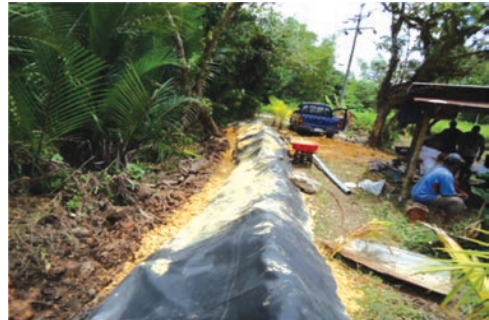
Fig. 80. Increasing the height of the main dike behind the summer house in Ngimis, Ngatpang
