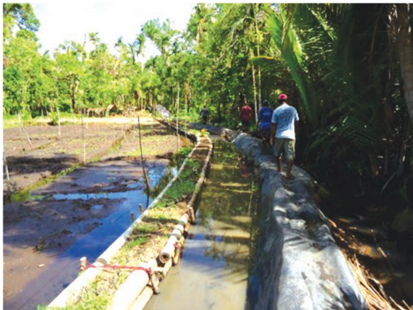
Fig. 84. Secondary dike constructed to protect the mesei in Ollei, Ngarchelong
